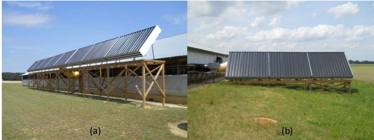
Figure 1. Solar duct at (a) turkey brooder farm in Snow Hill and (b) swine nursery in Roseboro, NC
